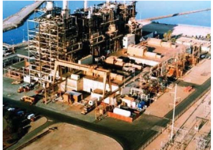
Chula Vista Power Plant
