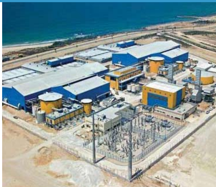
Ashkelon Desalination Plant
